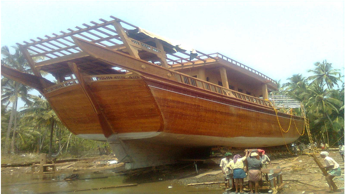
Launching Process (Source: Photograph by Researcher)
