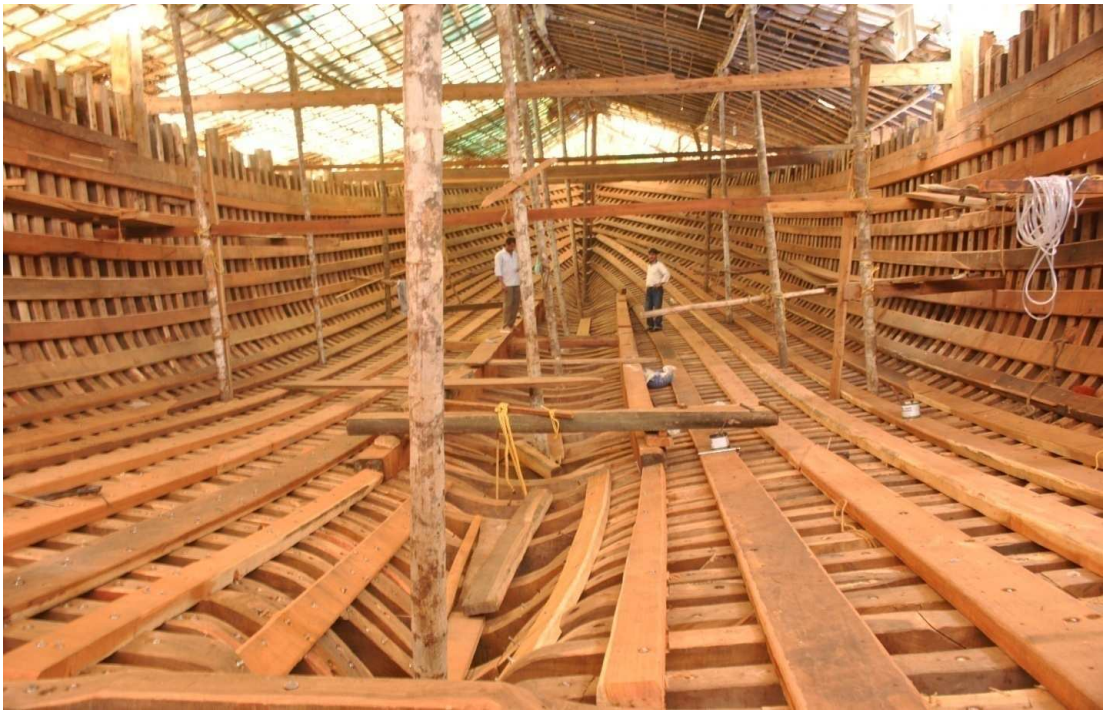
Interior Work (Source: Photograph by Researcher)
