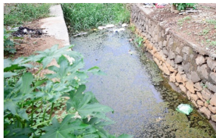
Blocked drainage
